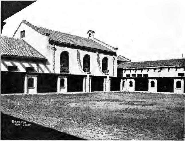
PATIO, EMERSON SCHOOL, OAKLAND
